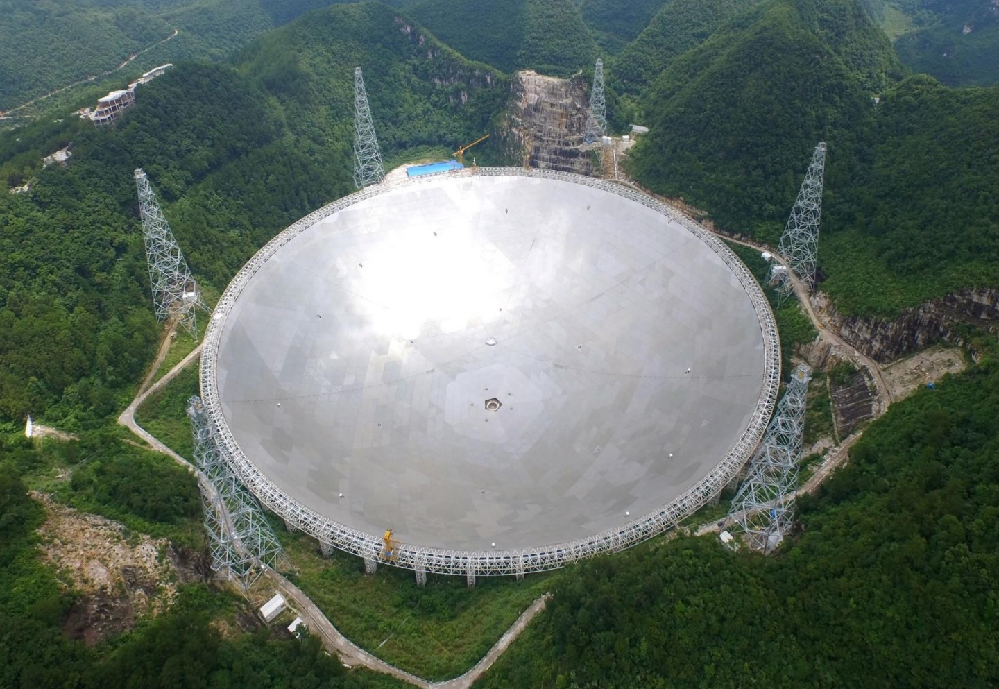
Largest Filled Aperture
