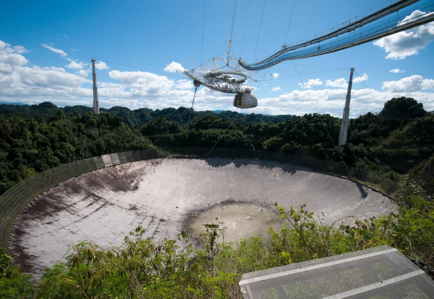
Largest Filled Aperture
