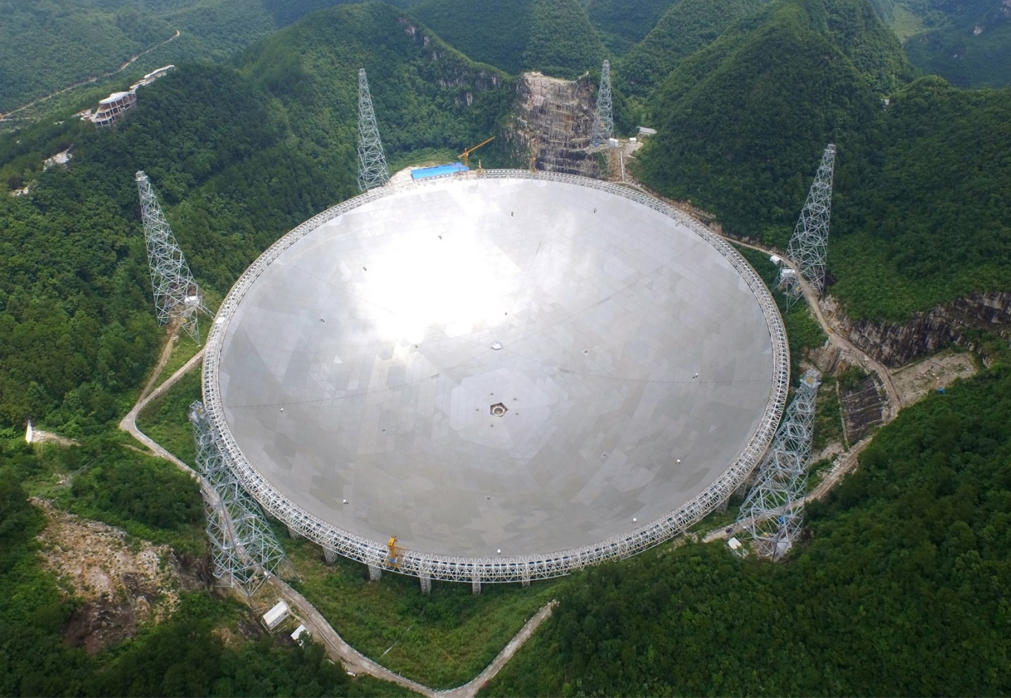
Largest Filled Aperture
